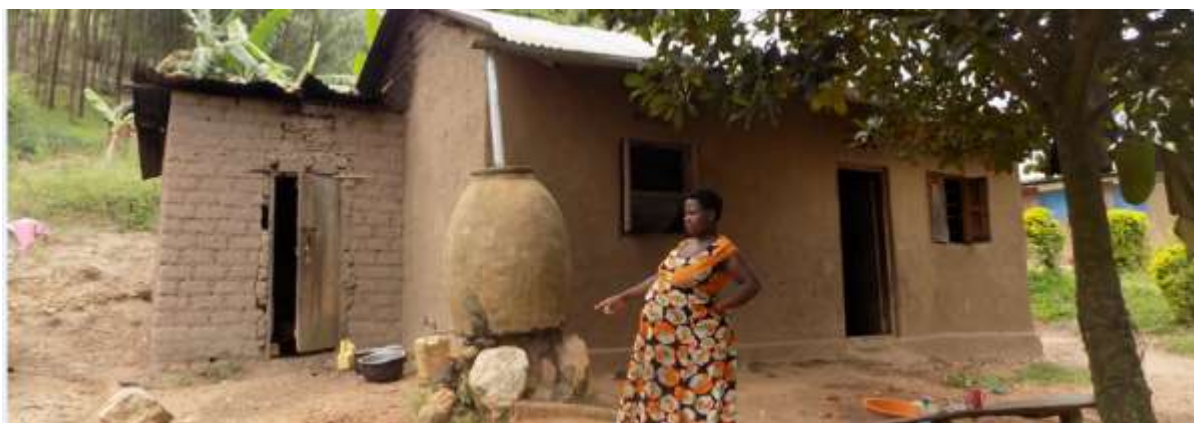
Figure 4-71: Rain water harvesting tank in Kabuyanda
