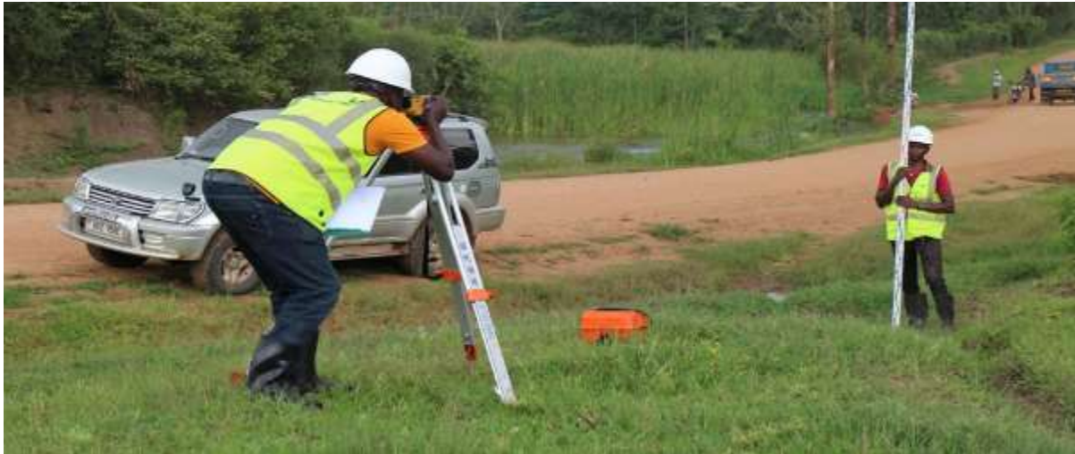
Figure 3-4: Picking the dry and wet profile cross-sections of Mishumba using a dump level set
