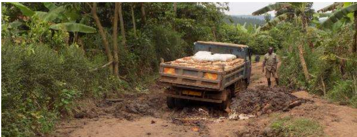
Figure 4-63: A truck stuck in mud due to poor state of roads during the rainy season at E233053, N9899555
