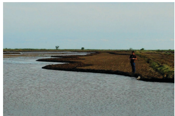
PHOTO A2.8 Contour Bunds Constructed with Highly Sophisticated Laser-Level Machinery
