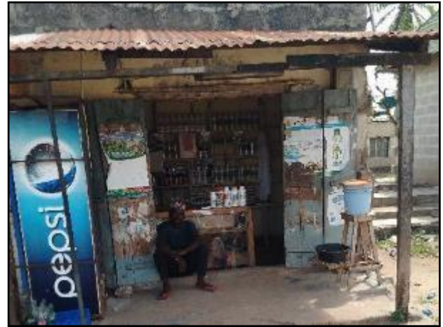
a) Example of Fixed Structures of Brick Walls, Concrete Foundation and Corrugated Iron Roofs
