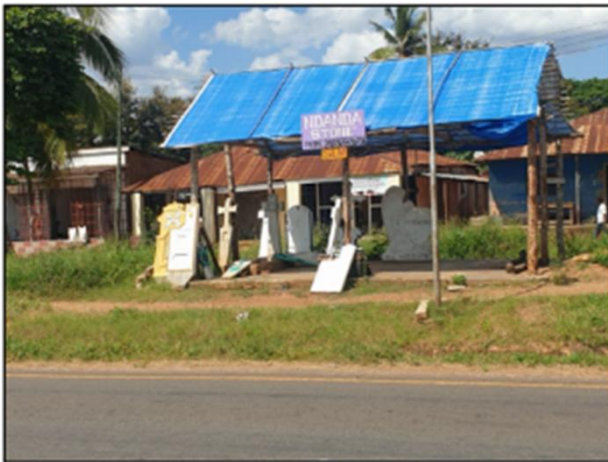
b) Semi-Mobile Structure of Wood Poles, Mixed Foundation and Corrugated Iron or Tarpaulin Roofs
