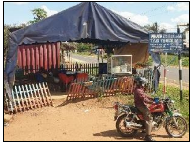
b) Semi-Mobile Structure of Wood Poles, Mixed Foundation and Corrugated Iron or Tarpaulin Roofs
