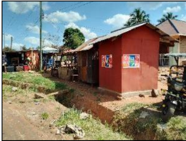
a) Example of Fixed Structures of Brick Walls, Concrete Foundation and Corrugated Iron Roofs
