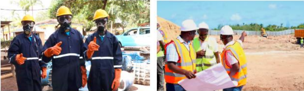
Right: Ongoing construction of fecal sludge treatment plant, Malindi.
