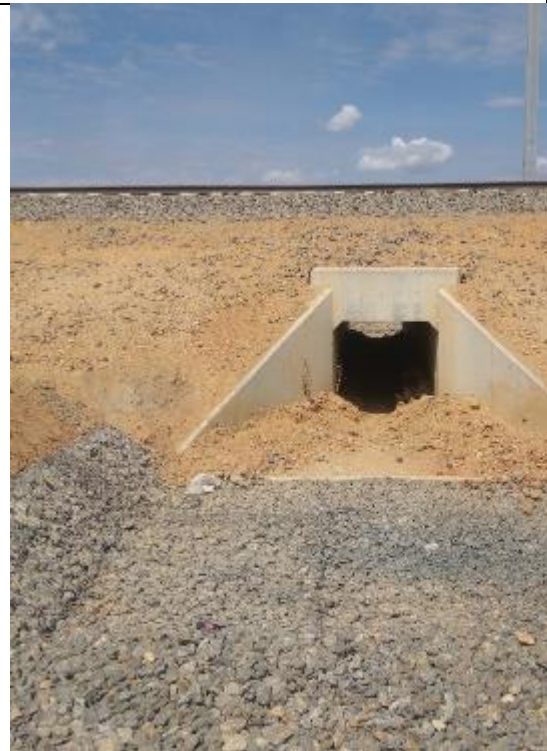
Well-packed Gabion Mattresses at Chainage 274 +634
