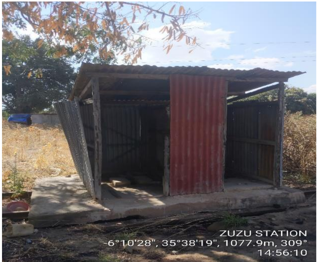
Figure 2.11: Toilet at Zuzu station
