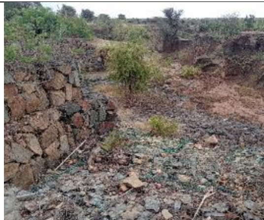
Gabion Boxes and Mattress Protections on Outlet of Culvert at Ch. 32+375
