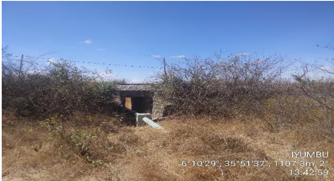
Figure 6.2: Water supply pipe crossing the project site at Iyumbu
