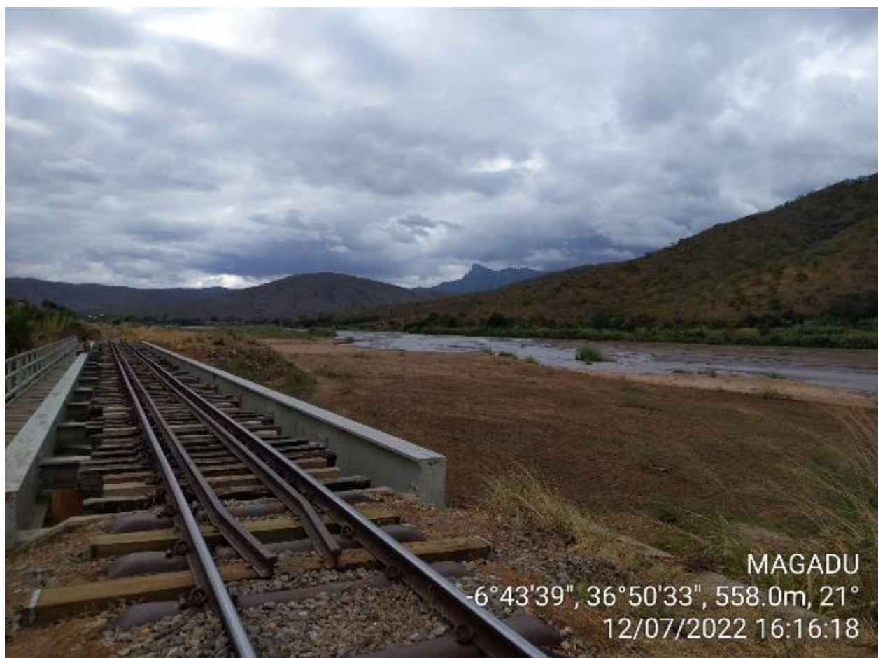
Figure 2.7: Wooden sleepers at Magadu
