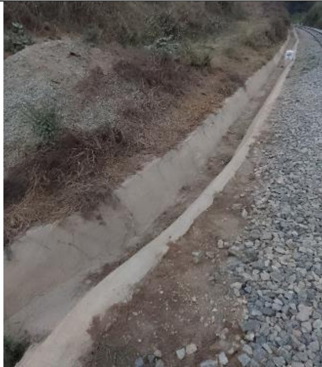
Small Open Rectangular Concrete Drain approaching Kilosa Centre at Chainage 281 + 870
