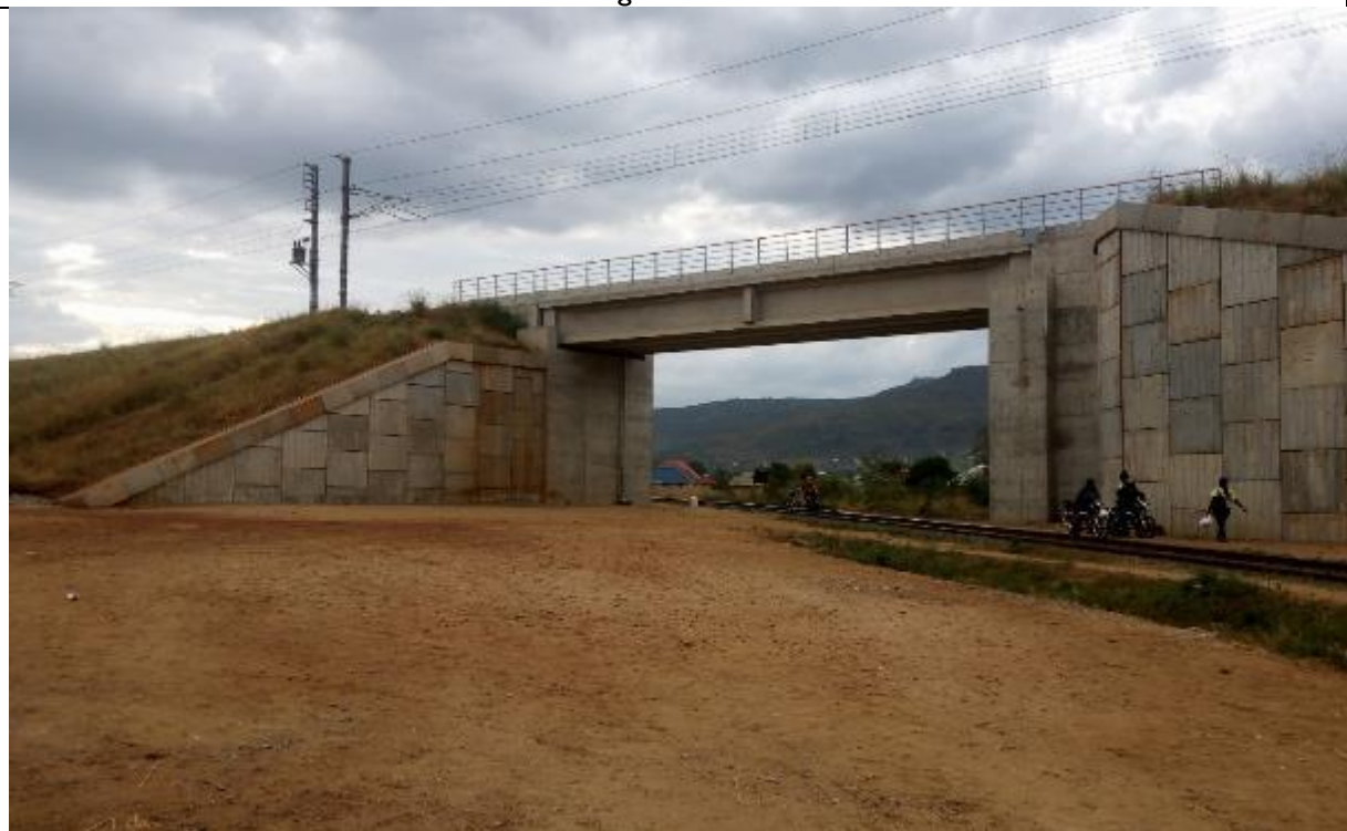
SGR Overpass Bridge at Lukobe (Morogoro Urban). at Chainage 230 + 201
