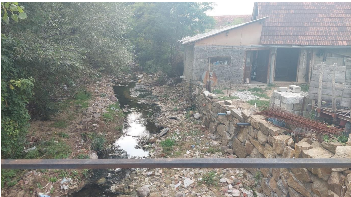
Typical site condition
