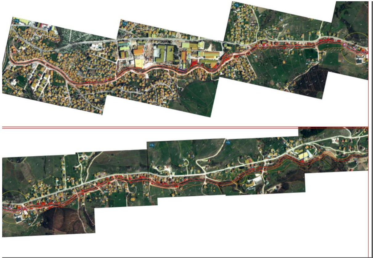
Figure 3 – River training works starting point from the mouth with Jošanica river
