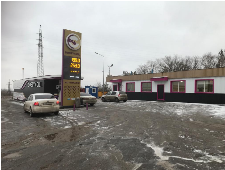
Figure 12: Gas Station and Car Wash
