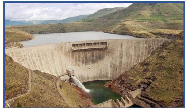
Souapiti Hydroelectric Power Plant (450 MW)
