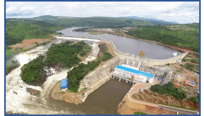
Kaletá Hydroelectric Power Plant (240 MW)
