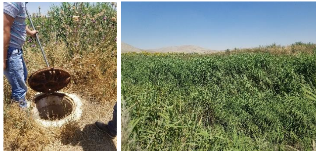
Figure 2.5 Existing Final Manhole and Discharge Point (will be the discharge point of Ilgın WWTP as well)
