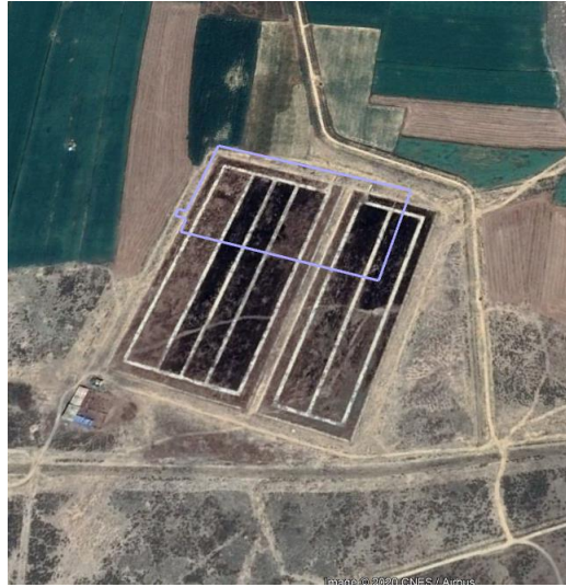
Figure 4.22 Satellite View of Stabilization Ponds and Project Site
