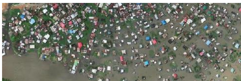
Figure 4.3. Aerial view flooded homes in Clara Town during the rainy season
