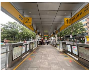
Fig 17: Bus station of BRT Line 1
