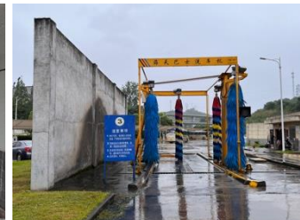
Fig 12: Vehicle washing site of bus depot
