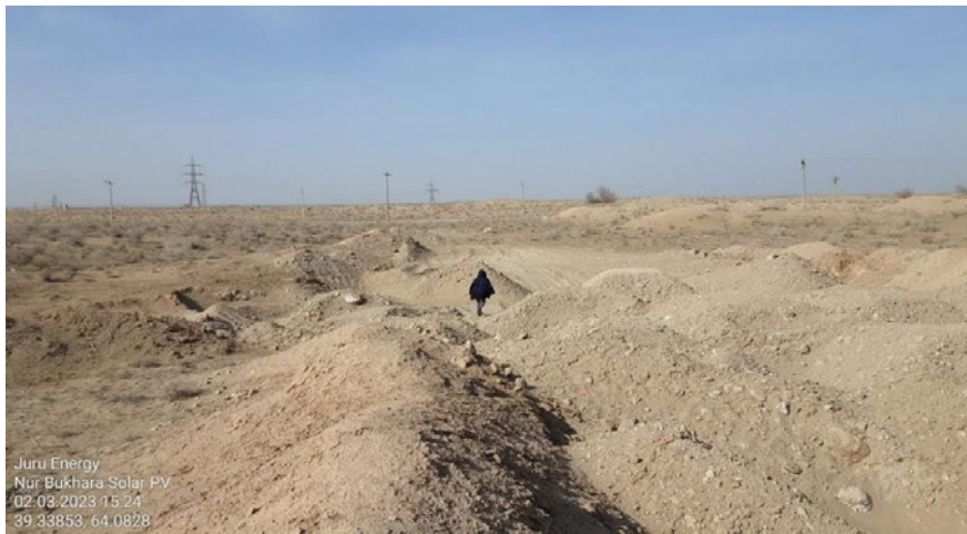
Figure 4: Excavations in the former quarry area
