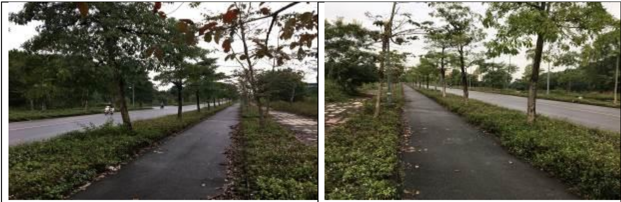
Rainwater drainage system is built submerged on the pavement
