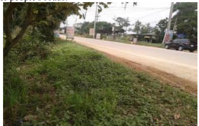
Figure 2.7: Existing Status of National Highway 21A
